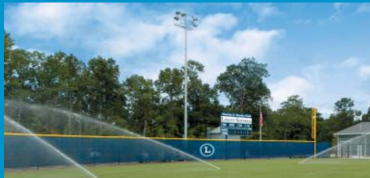
Much of the irrigation water required to irrigate Lovett School's two new sports fields comes from captured rainwater.
