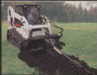
Track loader with Bobcat trencher.
