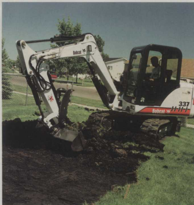
Subcontractors are often chosen for their expertise in a particular task.
