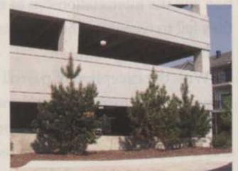
Maintenance will be easy here.
