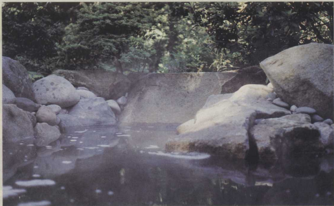
Schraven designed this spa, which is gunit and lined with boulders. It includes seating areas and jets to keep water moving.
