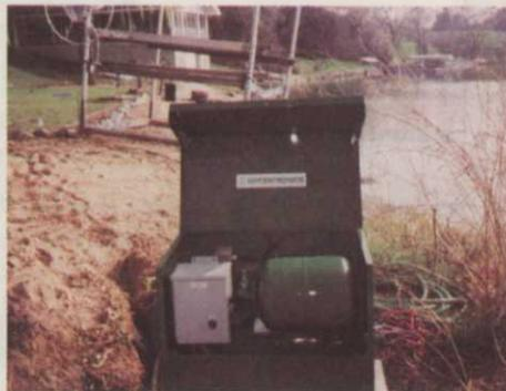
**This 7.5-hp pump station distinguishes between high-flow and low-flow pressure demands.**
