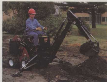
Toro SiteWork Systems with backhoe
