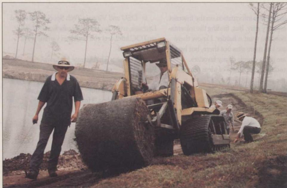
**A Posi-Track crawler conquered the landfill's 3-to-1 slope and saved more than 1,000 hours of handwork as it laid big-roll sod over a towering Florida landfill.**
