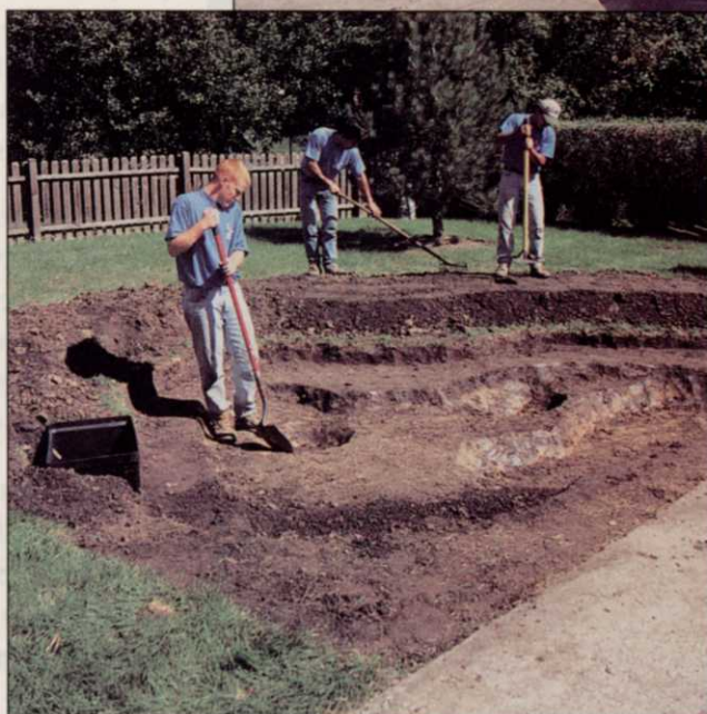
Left: once the pond site size is determined, remove the sod and dig out the pond.
