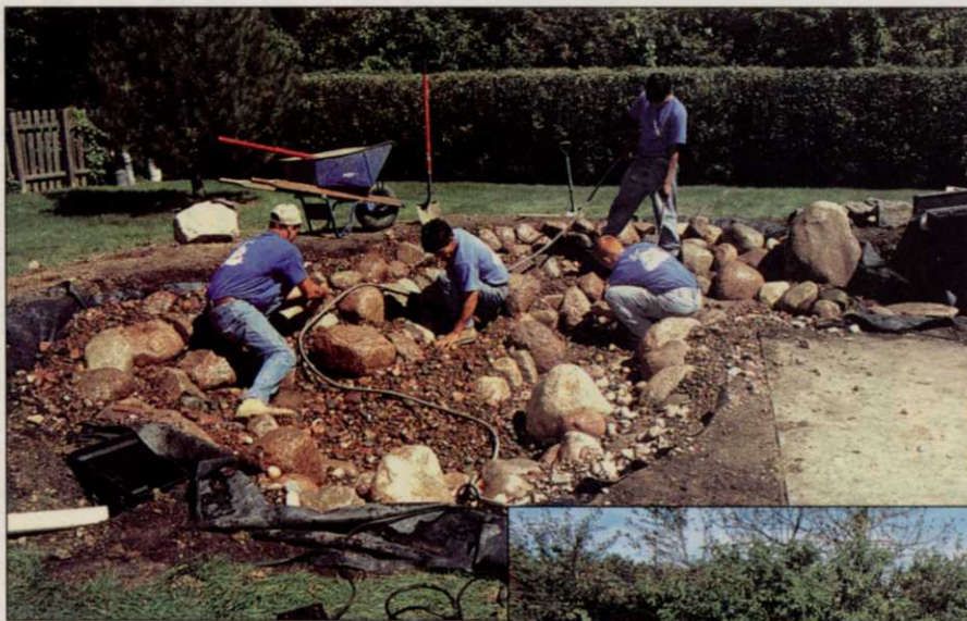
Left: wash off the rocks by using a garden hose while washing the dirt into the sump pump at the bottom of the pond. Bottom: Two or three tons of cobblestones are used around the berm for support. (Photos courtesy Aquascape Designs)
