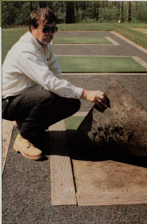
Concrete under each mat keeps the mats from getting that spongy, sinking feeling. Drain pipe runs under each slab.
