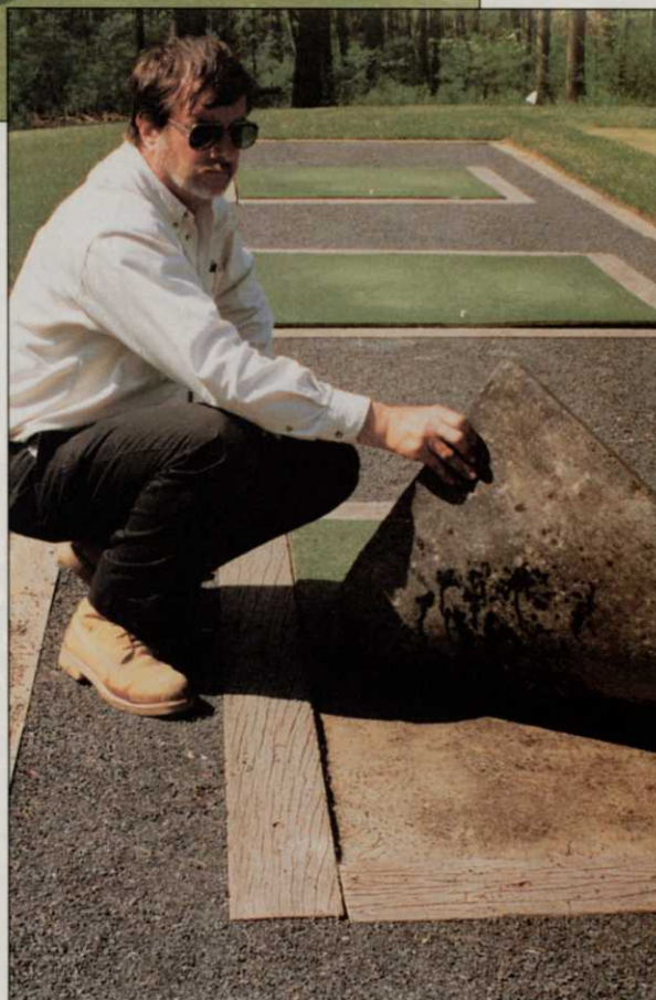
Concrete under each mat keeps the mats from getting that spongy, sinking feeling. Drain pipe runs under each slab.
