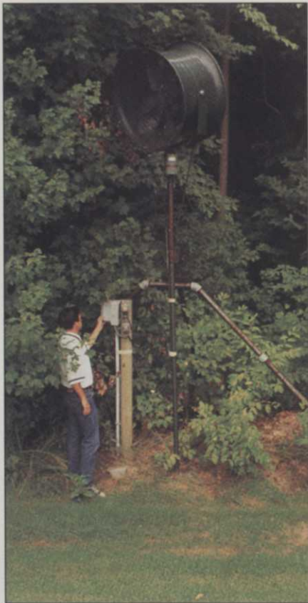
The fans at number 10 green circulate air and reduce chance for disease. Trees were reduced by 20 percent around this green. Fans by Paterson Fan Co., Blythewood, SC.
