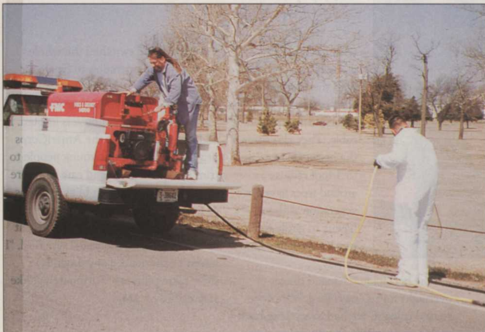
Spray technician, Charles Whitlock, applies the herbicide to the roadside as fellow technician, Kevin Johnson, attends to the sprayer.
