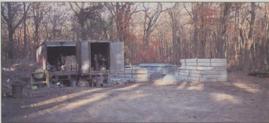
The staging area, where irrigation construction materials are held for use. Keep it organized.
