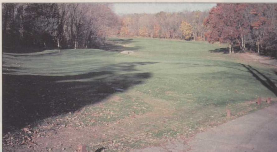
The main line and laterals are in, the area is cleaned up and seeded.
