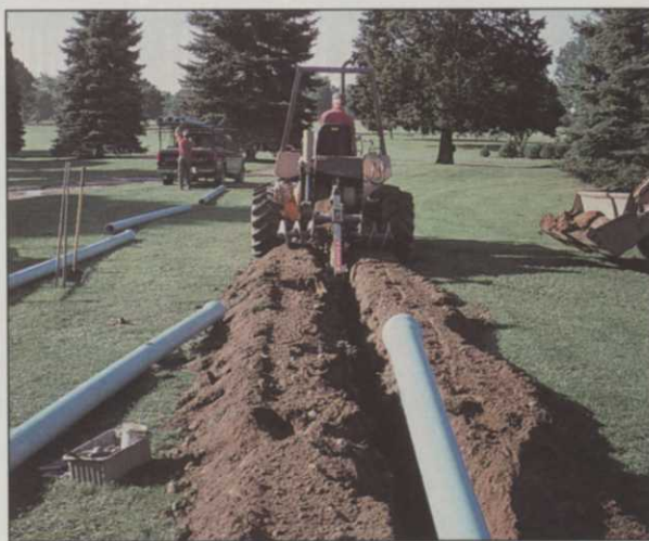
Lateral pipe and wire are installed with vibratory plow.
