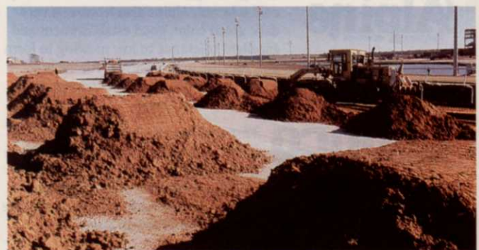
TurfGrids, fibrillated poly fibers, blended into this 80/20 planting medium provide stability to the bermudagrass racing surface.
