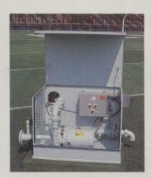
Ohio, also offers a line of self-contained single pump systems in a range of sizes. This line of pump stations, called RCTT (for Residential/Commercial Turf Tender) is powered with motors up to 30 hp with capacities reaching 300 gpm.
