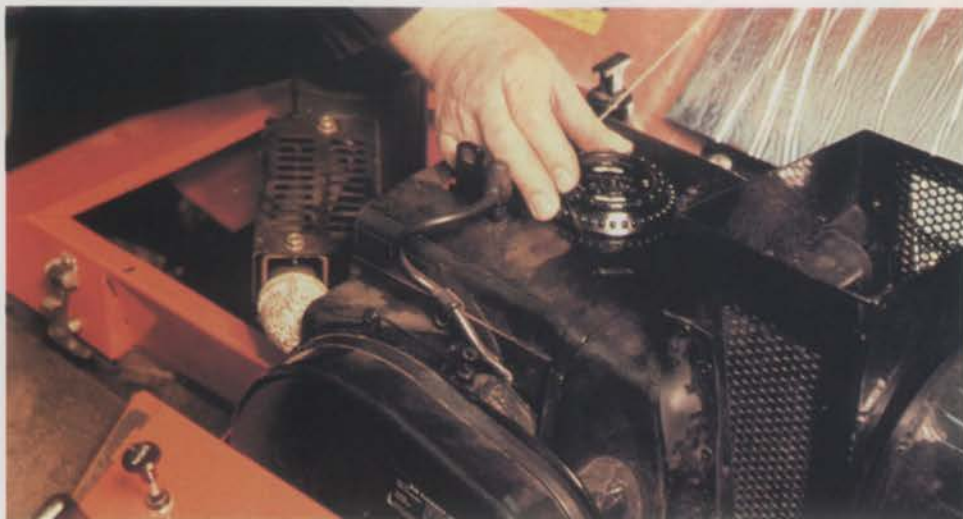
Equipment care is especially crucial in light of high equipment costs.
