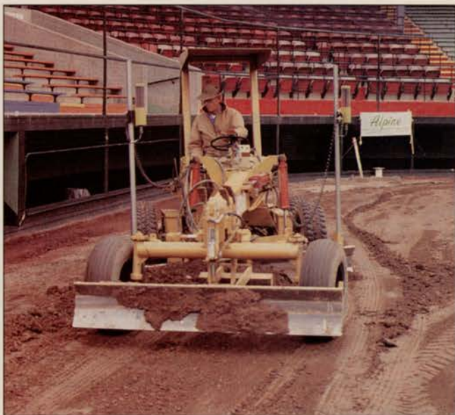
Grove Teates of Alpine Services used a laser to make sure Little League's World Series field drained to the warning track, foul lines.
