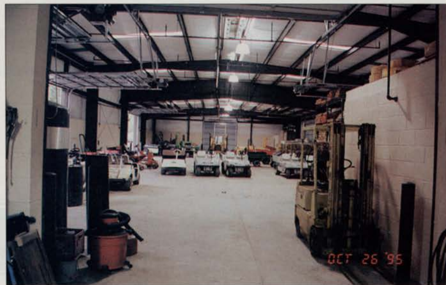
Finished. The new facility at Westchester includes a 2500 sq. ft. repair shop and a 6500 sq. ft. equipment storage area.
