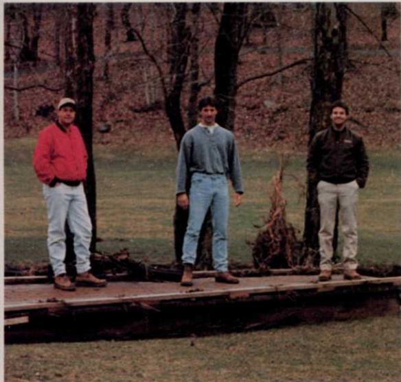
Mark Wilson's Valhalla crew made bridge repair a priority.
