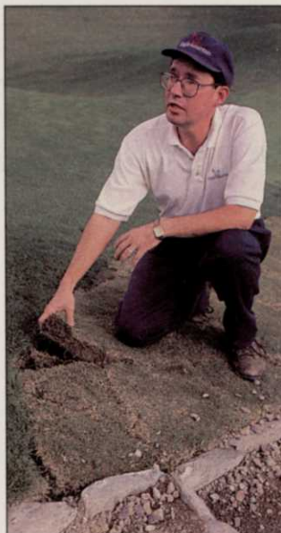
Smith has installed about 1000 square feet of artificial turf, and applied an athletic mix called Redi Play.
