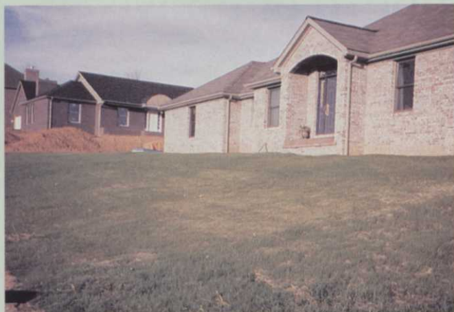
The North American Green reinforcement mat solved an erosion problem in this sloped lawn.
