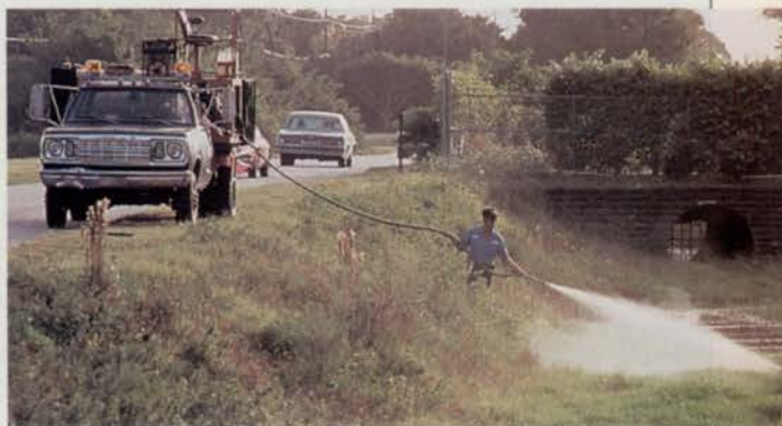
A worker applies Rodeo to brush growing in a roadside canal.
