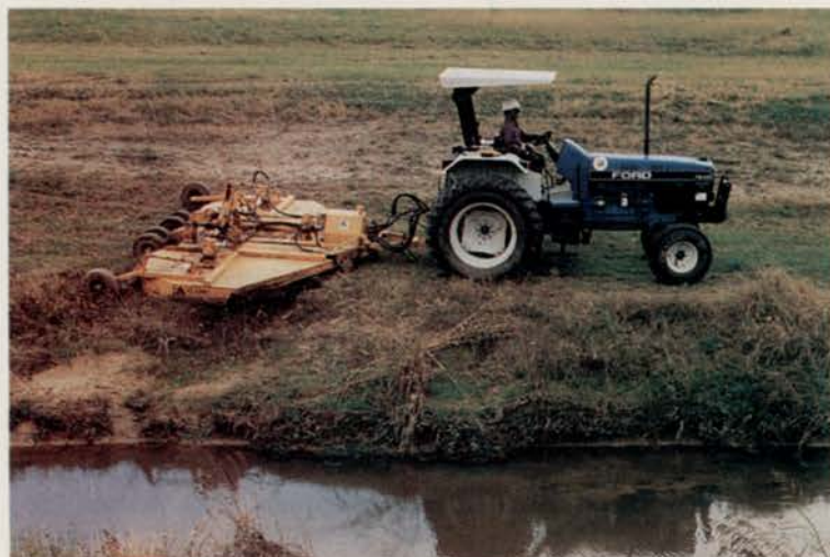
A 15-foot mower clears vegetation along flood control drainage canals.
