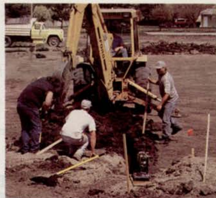
Four-inch perforated drain tiles were laid in 12-inch deep trenches.
