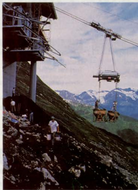
Topsoil and Alaskan mountain heather were transported both by tram (left) and by helicopter (right) to the area around a new tram station and support towers where the vegetation was to be transplanted.
