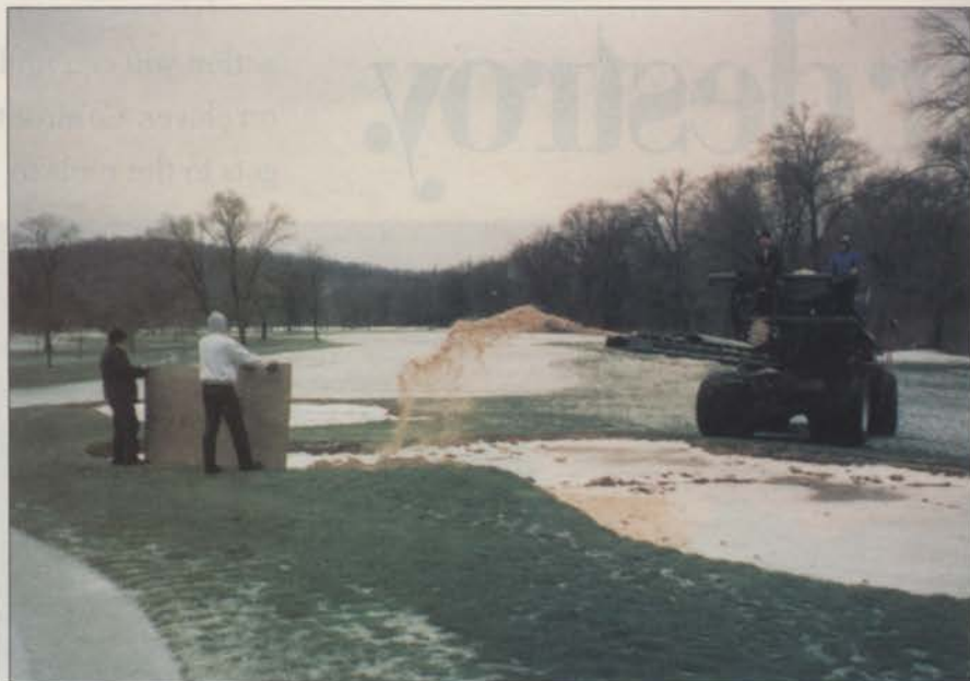
The swinging conveyor used for this job can fill a bunker in about 10 minutes. The tires exert a mere 9 psi of pressure on the turf.
