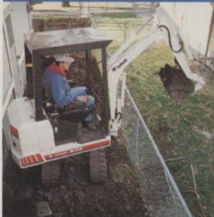
Replacing Drain Tile
