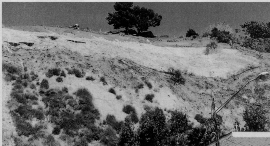
Poz-O-Cap, in the white area, was applied to a half-acre hillside in Malibu to prevent soil erosion.
