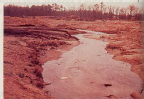
Stabilize pipe outlets with rock rip-rap or other suitable materials.
