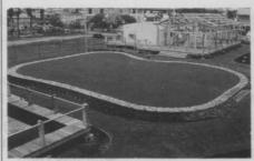
The surface features two inches of polypropylene filled with three types of aggregate fiber. It has a shock pad underneath with a simulated rootzone and vertical draining system.
