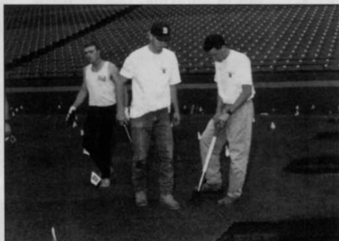
Some handwork is required to fit the hexagons into a nearly seamless 'pitch.'
