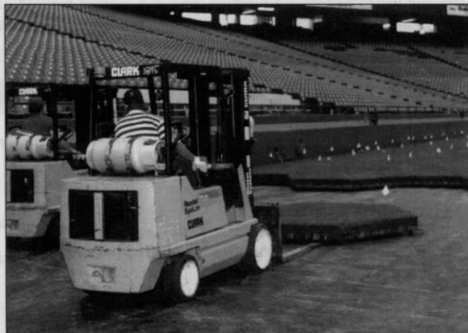
A fleet of forklifts positioned each of 2,000 separate pieces of sod into a rectangular carpet of turfgrass.
