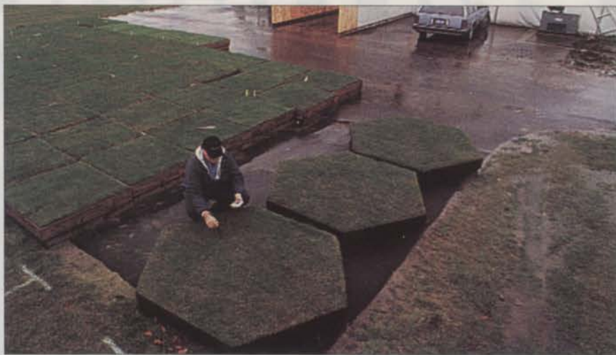
About 2,000 of these hexagonal turfgrass containers will be fitted together to make World Cup soccer field inside the Pontiac Silverdome. MSU's 'Silverdome West' in the background.
