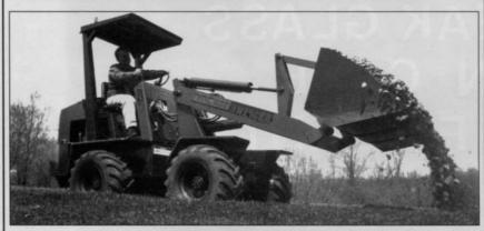
**Swinger** – all around turf and landscape loader has flotation tires and "no-scuff" articulated steering. Handles everything from rock to hay. 3 sizes available with lift capacities from 1,175 to 2,100 lbs. SAE rating. Has a variety of bucket sizes from 12 to 36 cu. ft. and single lever "joy stick" bucket control.
