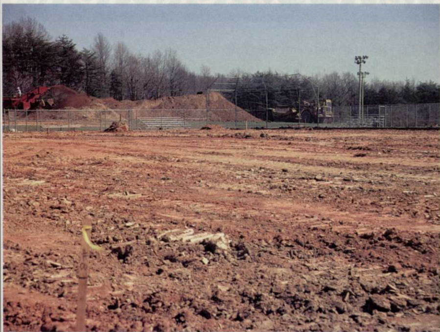
An athletic field after stripping and stockpiling of topsoil shows promise for the future.
