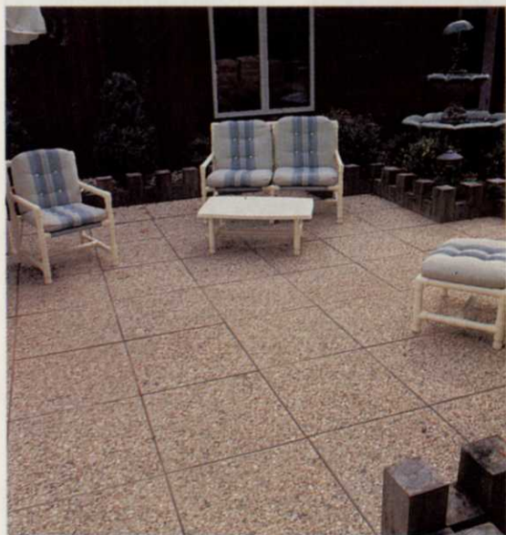
These Terra-Pavers, from Wausau Tile, can be installed over bituminous sand or mortar beds. They hold up well under pedestrian and moderate vehicular traffic.
