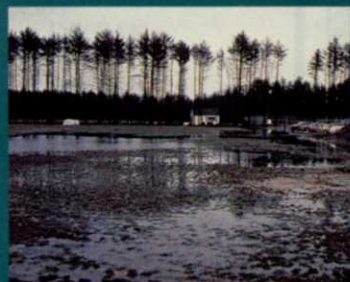
Somebody made a big mistake with this newly-constructed field when they did not allow for proper drainage.
