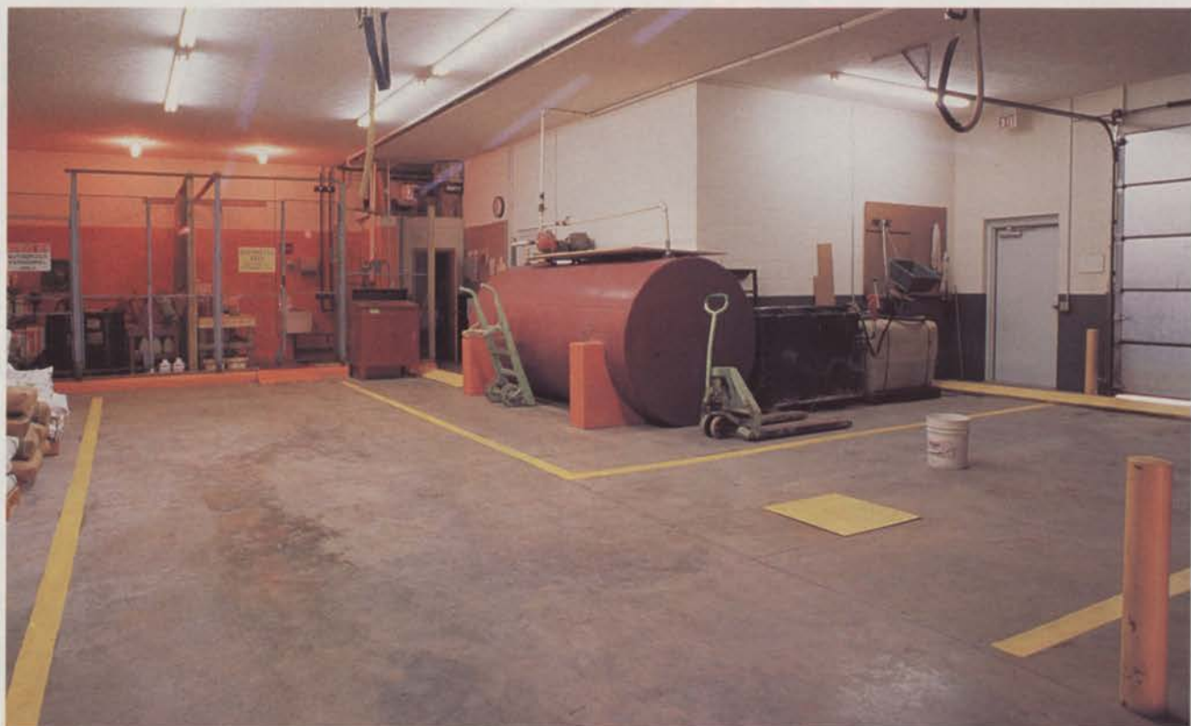
The secondary containment area is used for storage, parking and load-and-fill operations.
