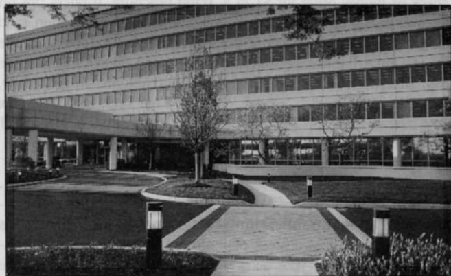
The Scott Paper Co., 'before-and-after.' The Brickman Group transformed a simple asphalt square into a parkway, enhancing visual impact.
