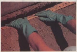
The Biobarrier system provides long-term prevention of root encroachment.
