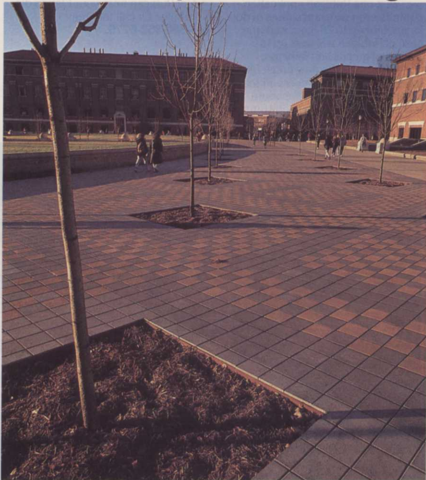
The stones used to pave Purdue Mall have a minimum compressive strength of 8,000 psi (photo courtesy of Mobay Corporation of Pittsburgh).
