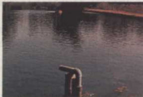
30 days after installation
