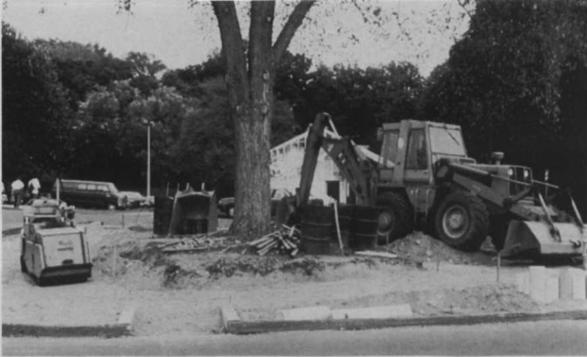
Construction remains one of the biggest threats to trees. Injuries are caused by raising or lowering of grade and by trenching near the tree. Still, injured trees may take years to die.
