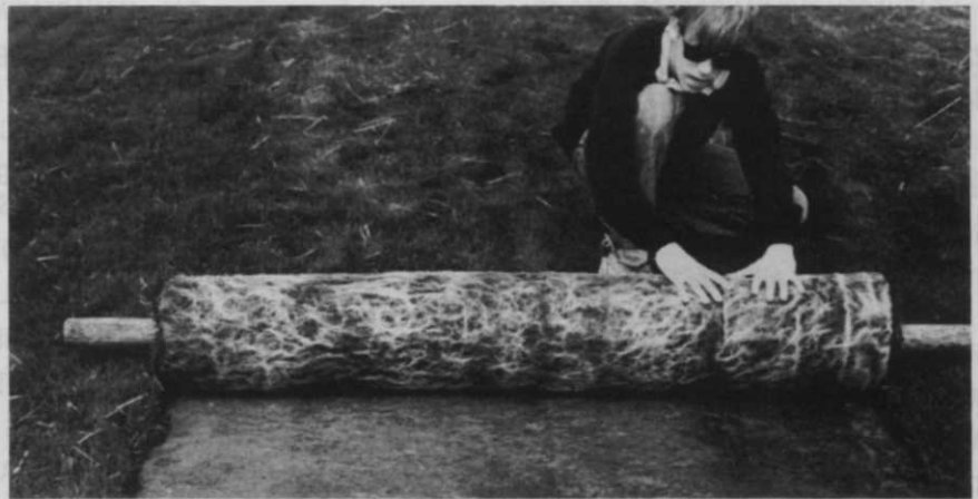
The availability of composted sludge and the arrival of tall fescues make the concept of growing sod over an impermeable base more feasible.
