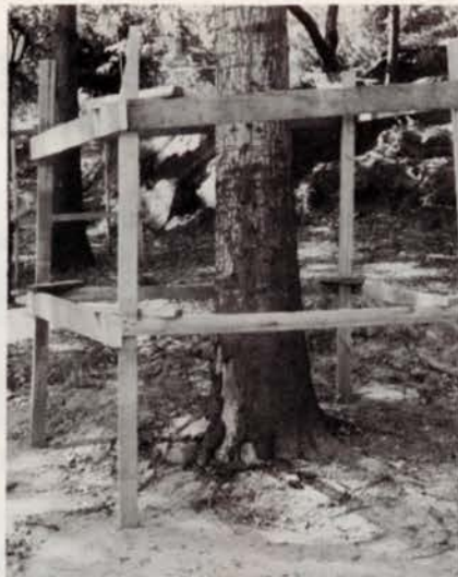
The "wooden cage" fails because it doesn't adequately protect tree roots.
