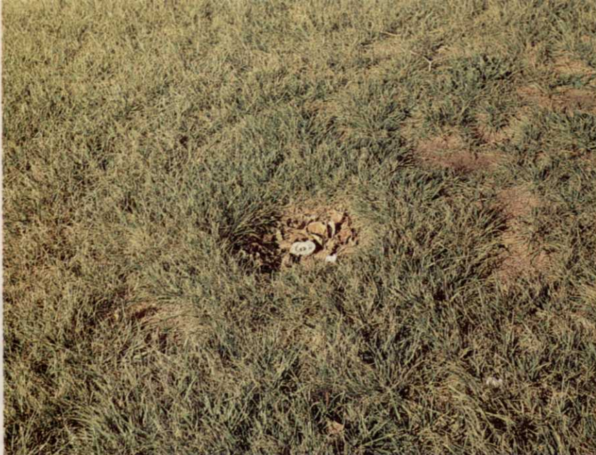
Irrigation heads should rise high enough to spray over the top of mowed grass. Grass scalped around heads with line trimmers is more susceptible to weed invasion.
