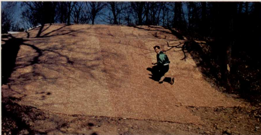
After seeding, erosion control blankets are installed.
