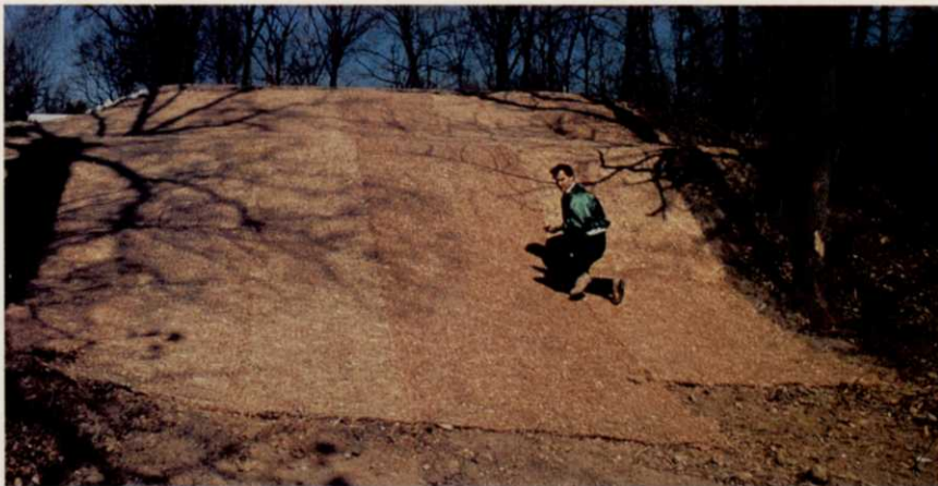
After seeding, erosion control blankets are installed.
