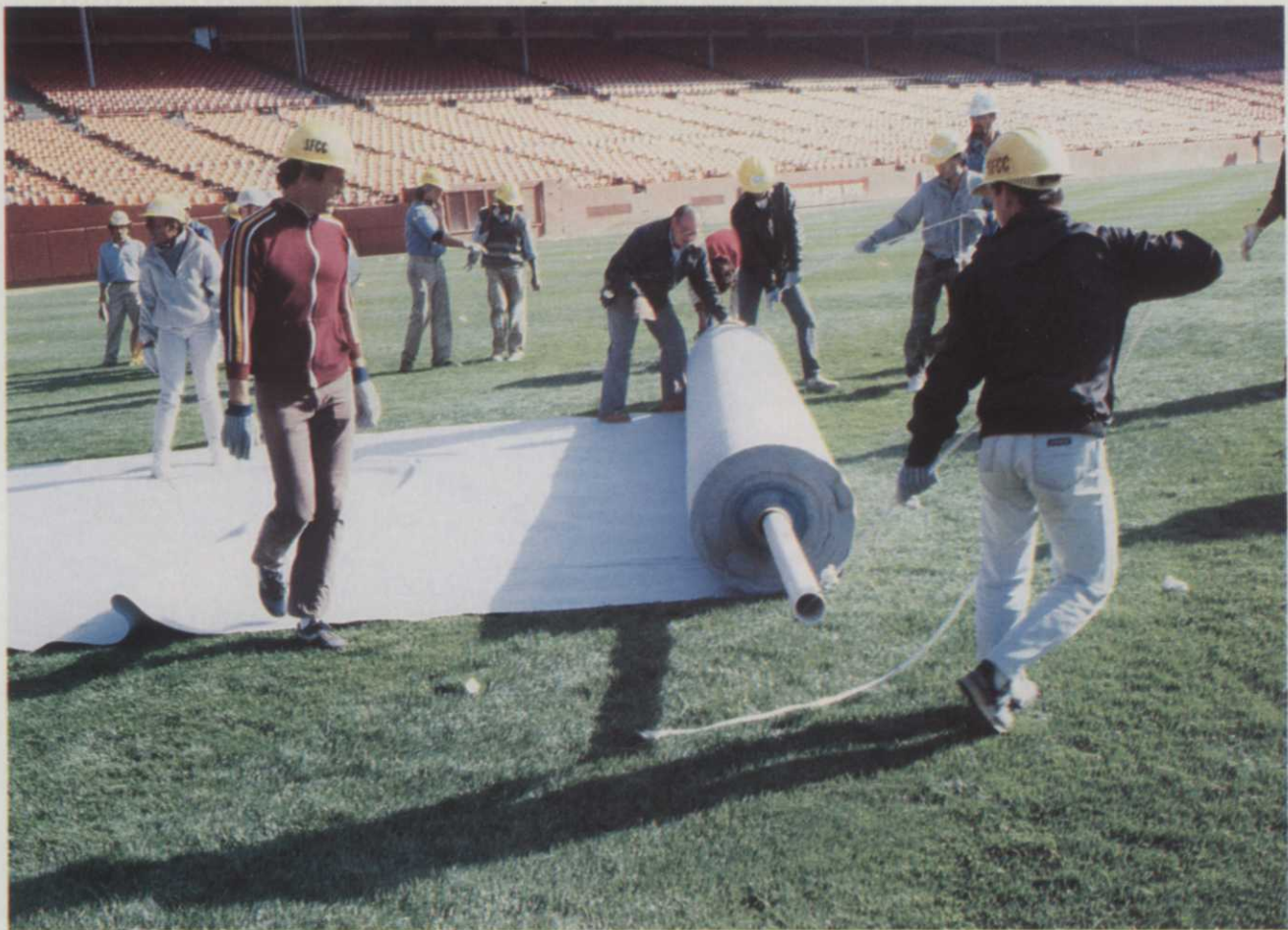
Candlestick's crew, along with volunteers, starts to unroll the TerraCover to protect the field against wear.
