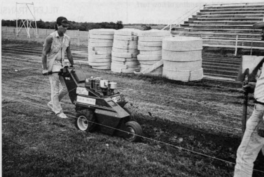
Digging the trench for the 12-inch TerraFlow trunk line along one sideline using the Ditch Witch 1010 trencher.
