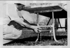
driving it into the earth to the proper depth, then wrapping the chain or cable around the drive rod and pulling upward, rotating the anchor into a loaded lock position underground. Use a padlock or other device to attach the chain or cable to the object being secured.
