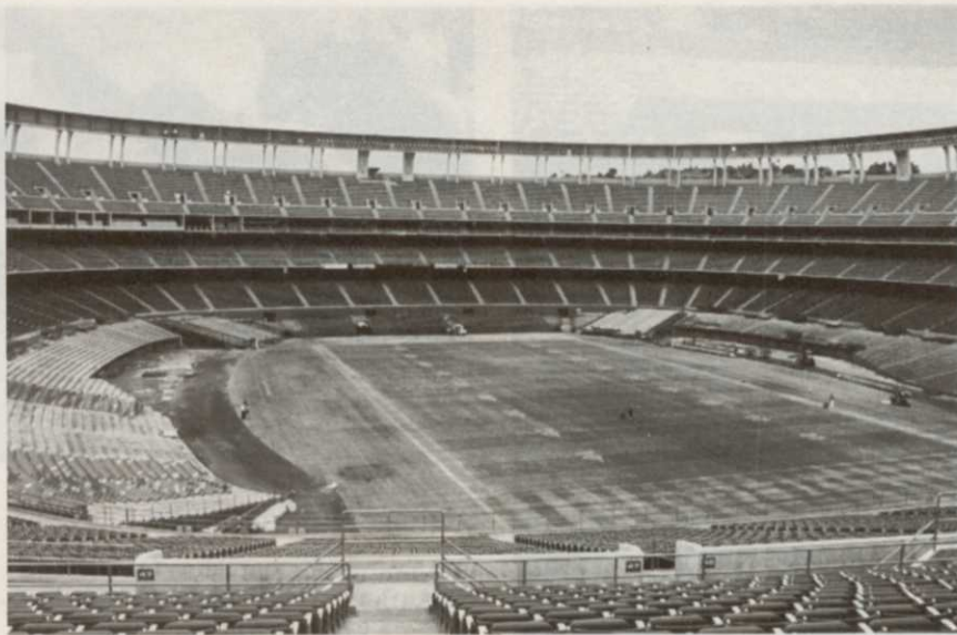
Jack Murphy Stadium before Toma's crew worked on it.
